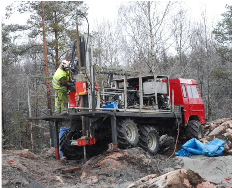
Figure 4.2 The core drilling machine that performed the drilling at all locations.
